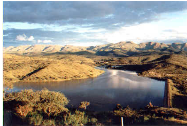
Figure 48 Avis Dam - incorporating nature into the city
