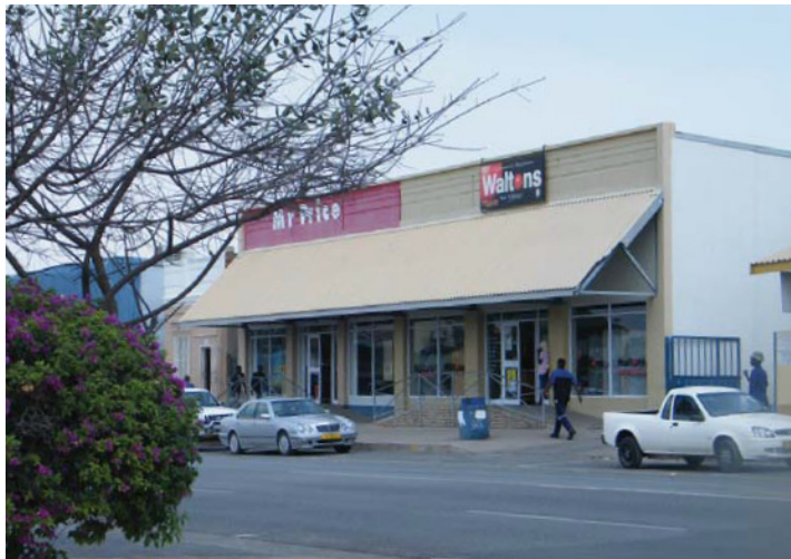
Figure 45: Newer buildings with shade structures
